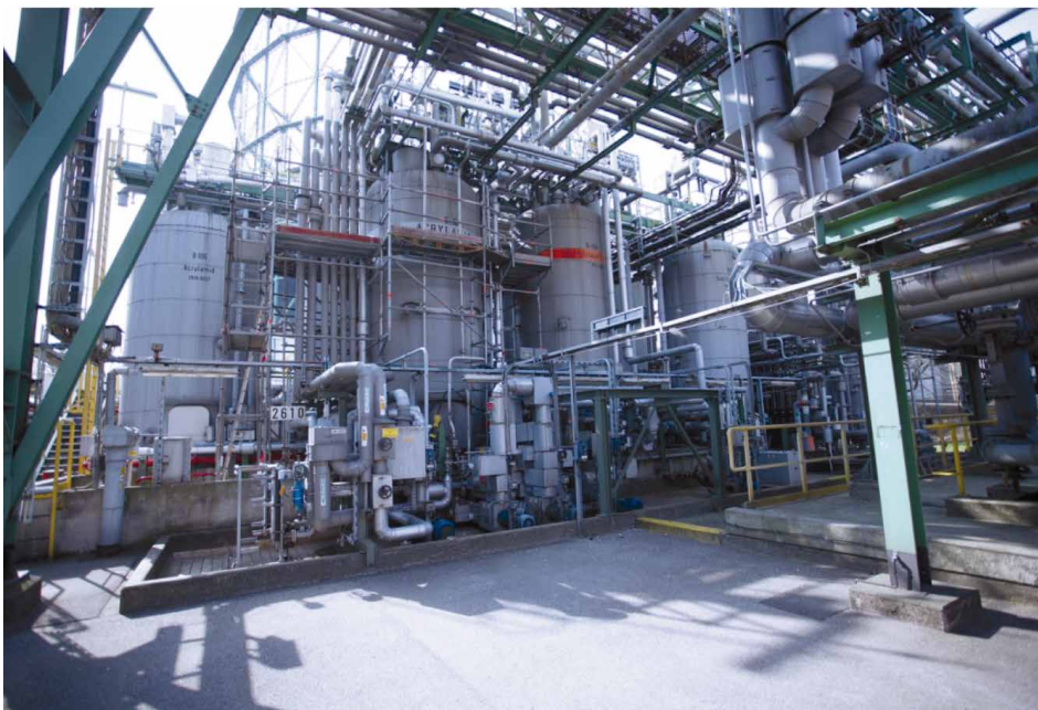
Photos by courtesy of MAN Diesel & Turbo SE
